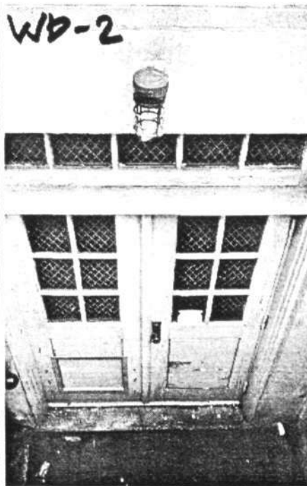
WEST DOOR #2 @ LOADING DOCK
