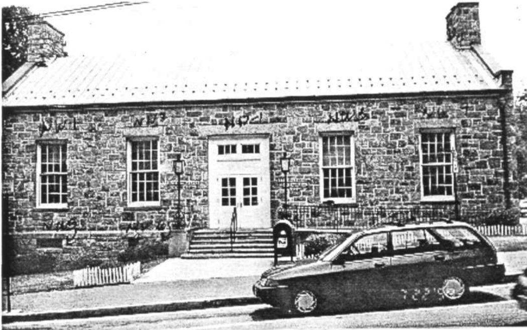
NORTH ELEVATION, MAIN ENTRANCE
