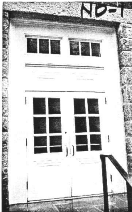
NORTH DOOR #1, MAIN ENTRANCE
