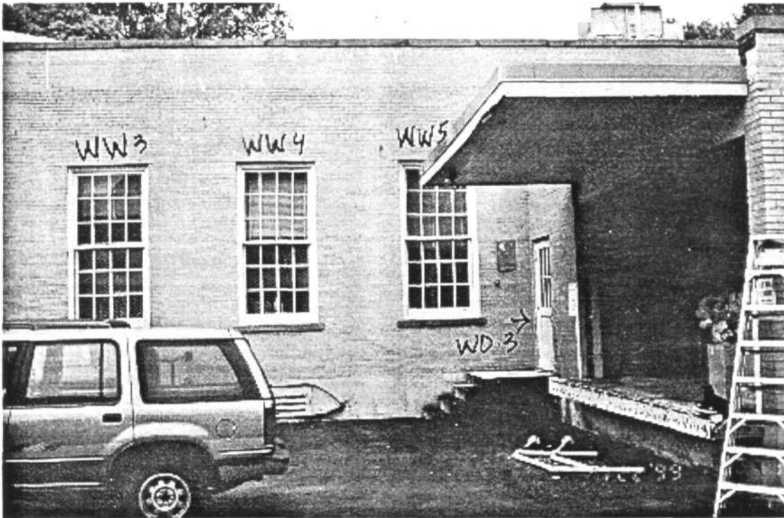
WEST ELEVATION, LOADING DOCK
